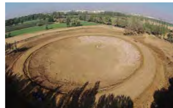
© Construction of an artificial lake, 15,000 m 3 – Start of works.
