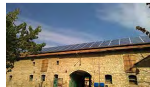
© Installation of a solar PV panels farm, 28.6 KW peak
