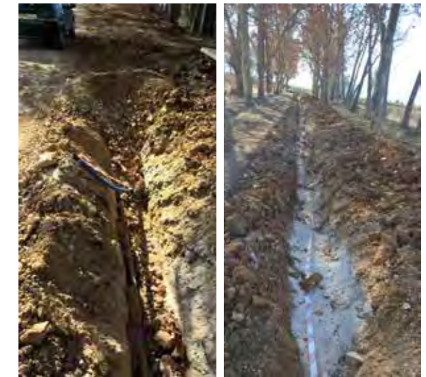
© Excavation and installation of a potable water network
