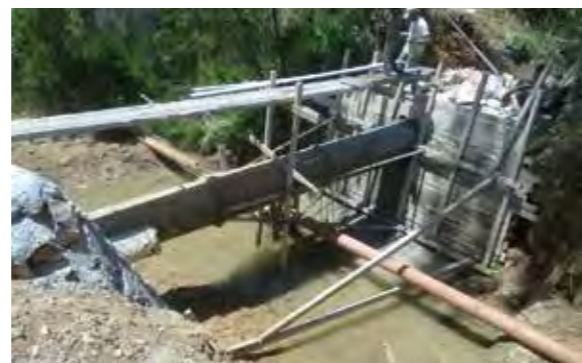
© The same water duct after replacement and building supportive walls.
